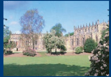
Auckland Castle – the 800 year-old seat of the Bishop of Durham and venue for the IBRU workshop dinner.
